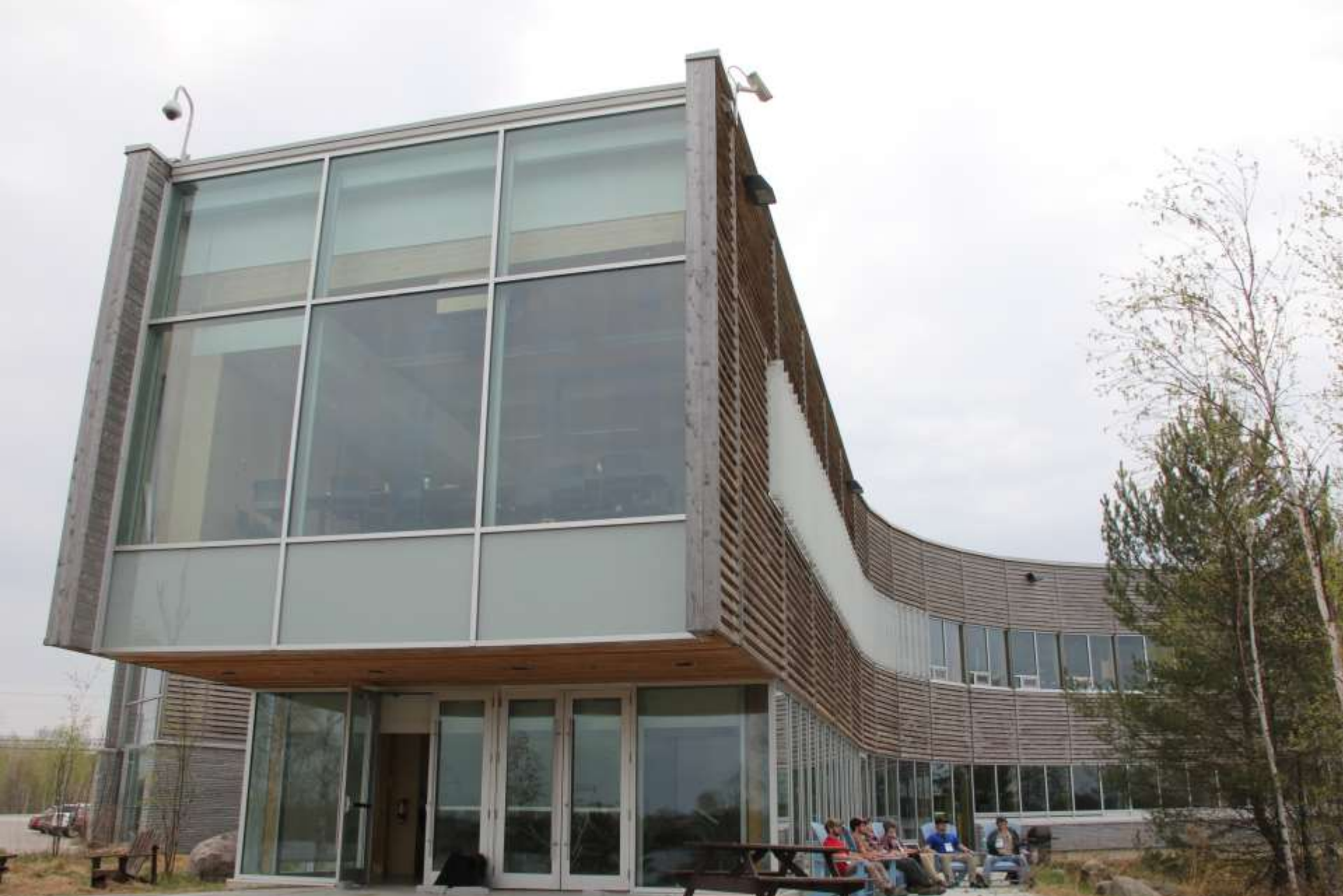
The beautiful Vale Living with Lakes Centre at Laurentian University, one of the most environmentally-
