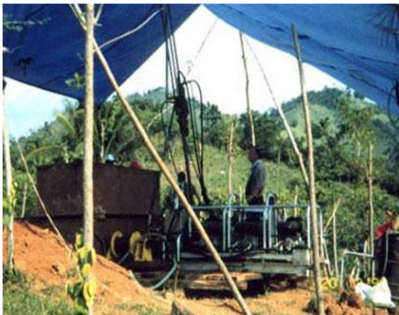
Figure 38: Lightweight, modular drill rigs can mitigate environmental disturbance in tropical terrain. © Kluane Drilling
