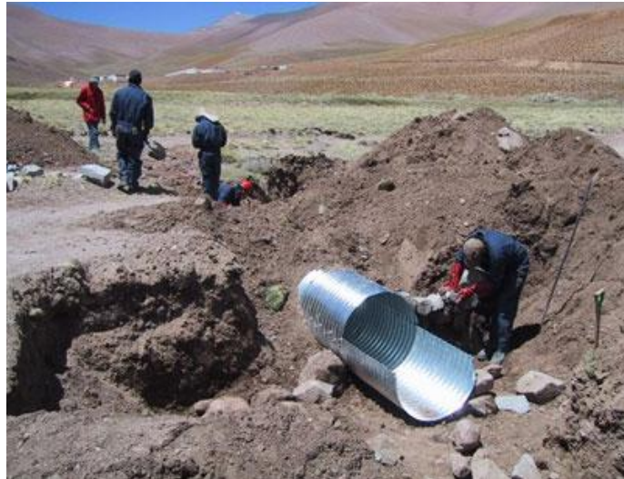
Figure 19: Placing a culvert in the high Andes of South America. © Noranda/Falconbridge
