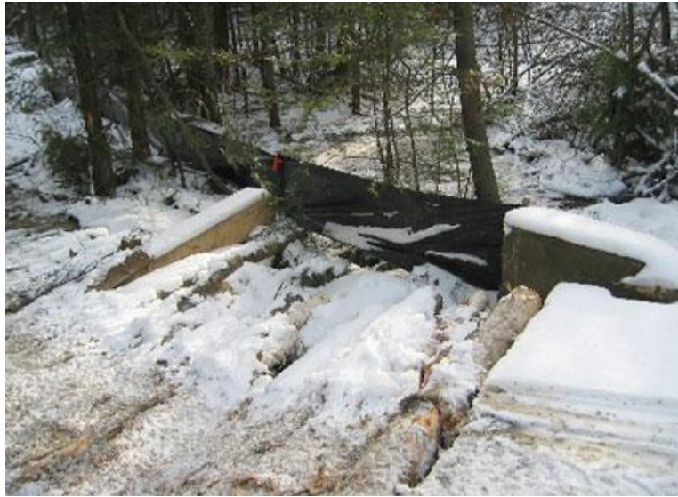
Figure 22: Silt fence in place on stream crossing in northern Canada. © Noranda/Falconbridge.
