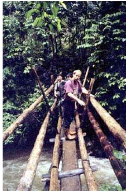
Figure 16: Bridges can be constructed from local materials and need not be major structures if equipment can be moved by hand as in this example from Central America. © Energold
