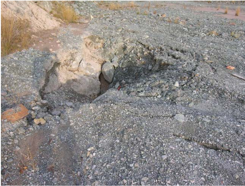
Figure 22.3: Slumping ground on the surface above underground mine workings © Courtney Mitchell
