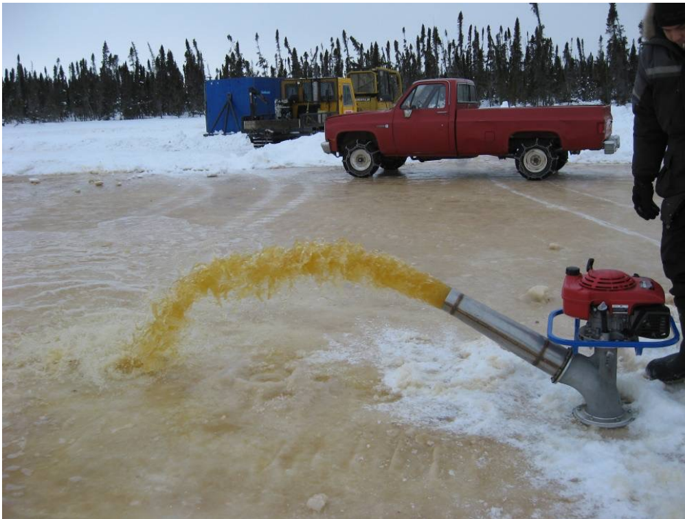
Figure 21.6: To create a thicker safer ice road, the ice is flooded to create "lifts" that freeze solidly within 12 to 24 hours. © Chris Pederson
