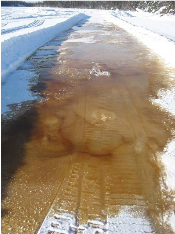
Figure 15.7: Overflow on a trail crossing a swamp © Jens Pedersen
