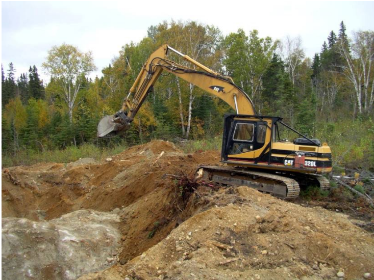
Figure 21.8: Pile the excavated material at least one metre back from the edge of the trench. © Lorne Burden
