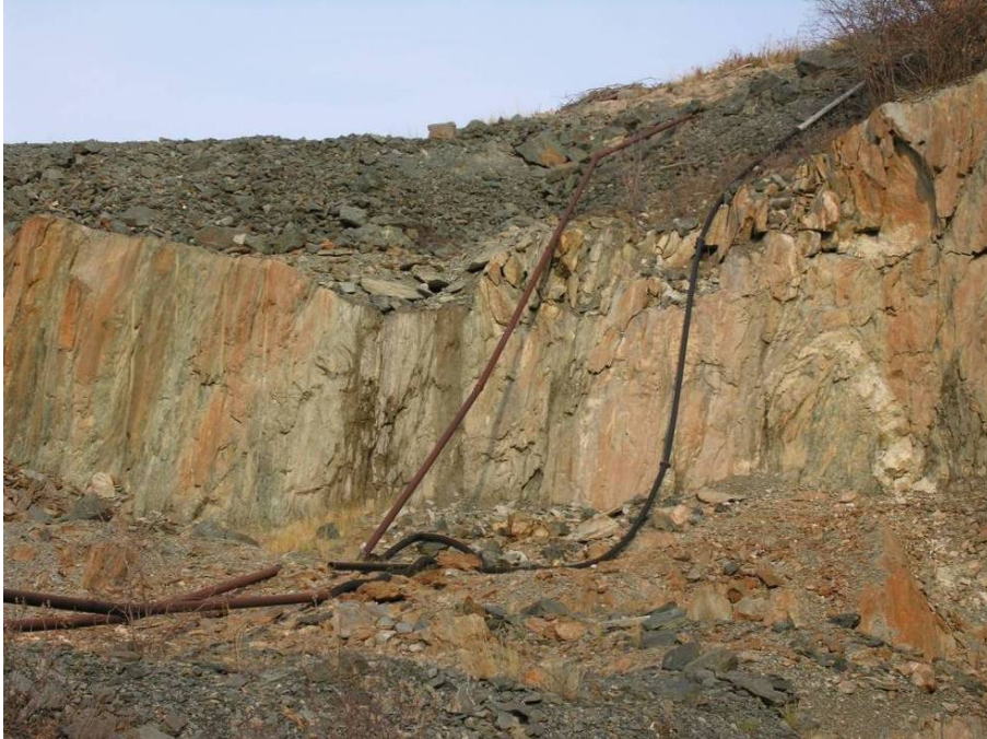
Figure 22.2: Unstable loose rock above a pit wall, dangerous footing, and a risky place to sample. © Courtney Mitchell
