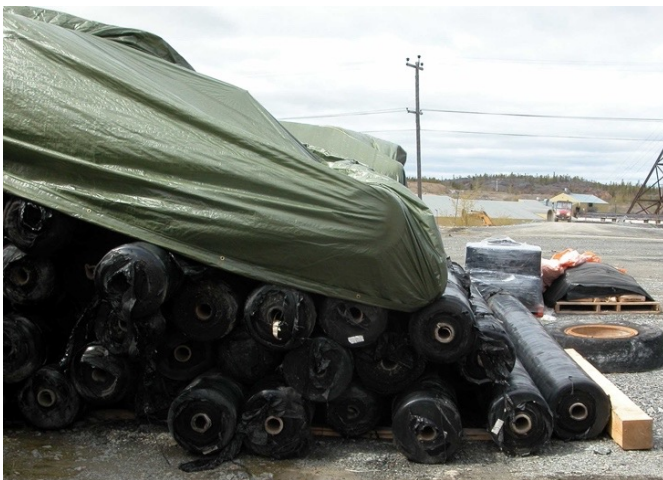
Figure 18.10: A dangerous pile of geofabric rolls: provide adequate end support to prevent collapse. © Courtney Mitchell
