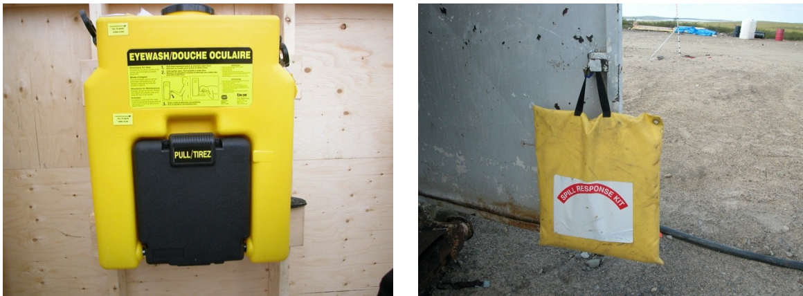
Figure 18.2 Site specific emergency response equipment: eye wash station (left) and spill kit (right). © Bill Mitchell
