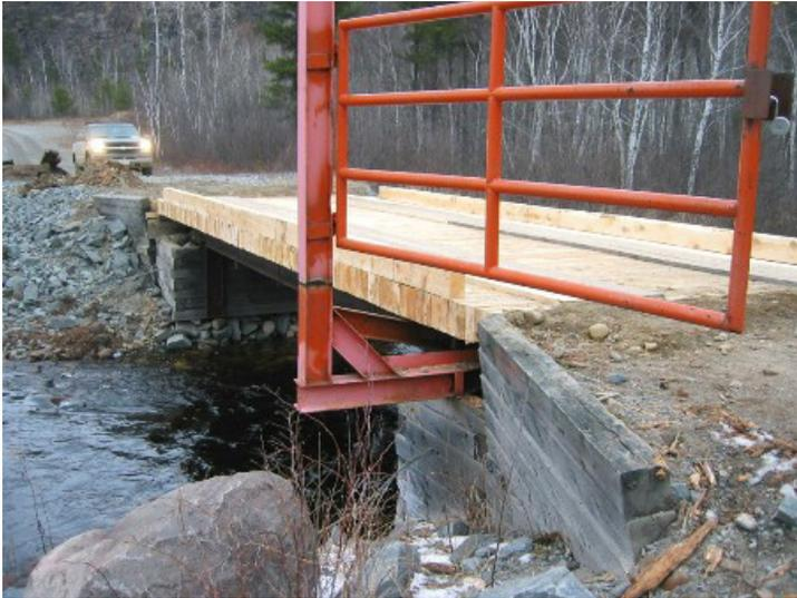
**Figure 18:** Good example of a steel girder bridge with wooden deck and stone-filled cribs. Locking gate can be used in this case to control access. © Noranda/Falconbridge
