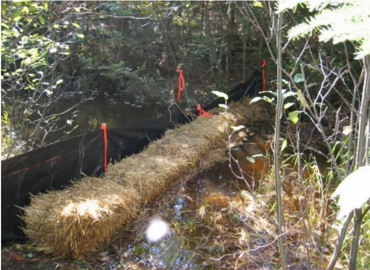
Figure 21: Used together, silt fencing and hay bales can be very effective in some circumstances. © Noranda/Falconbridge.
