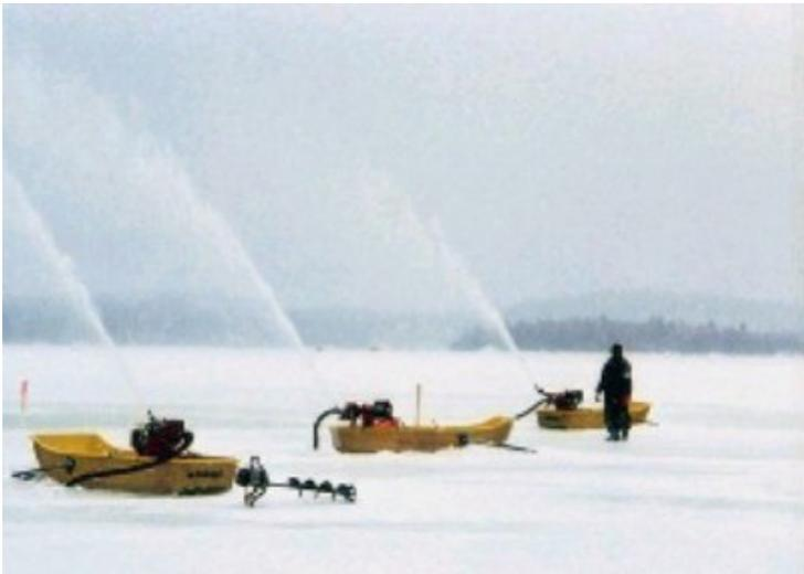
Figure 58: Building the ice pads on Windy Lake. © Wallbridge
