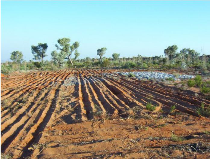
**Figure 34:** Scarifying by bulldozer of old drill site to assist in rain retention and encourage plant growth. South Australia. Photograph from Mithril Resources Ltd.
