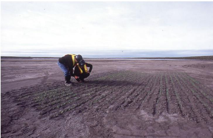
Figure 52: Reseeding an abandoned airstrip in the sub-Arctic with local hardy plants. © BHPBilliton
