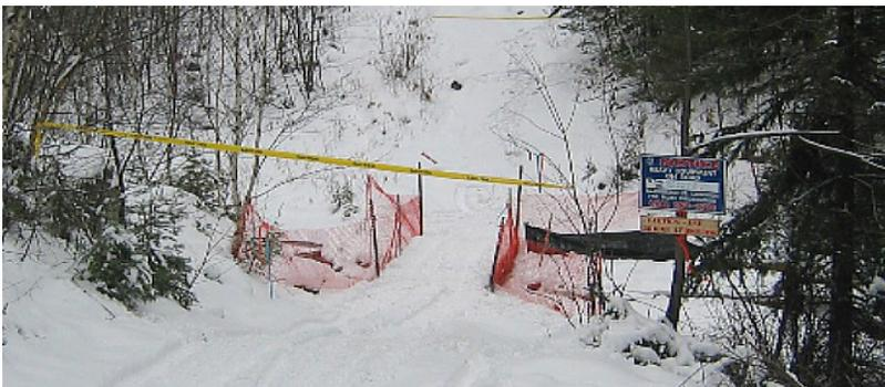
**Figure 20:** Winter stream crossing. Note use of snow fencing for guidance, warning signs and silt fencing. © Noranda/Falconbridge
