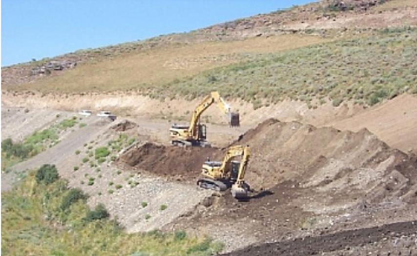
**Figure 66:** Road reclamation usually involves two excavators working in tandem. The original slope is restored by cutting down the upper slope and pulling up material from the lower slope. © AngloGold.
