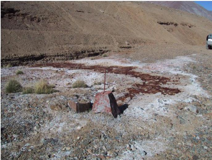
**Figure 48:** With proper capping and, if necessary cementing, seepage of groundwater with high metal content can be avoided. © Noranda/Falconbridge.
