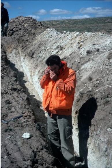
**Figure 11:** Trenching can leave a major scar on the landscape unless reclaimed. The muck pile from this trench in Argentina will be used as backfill upon completion of work. © lamgold.
