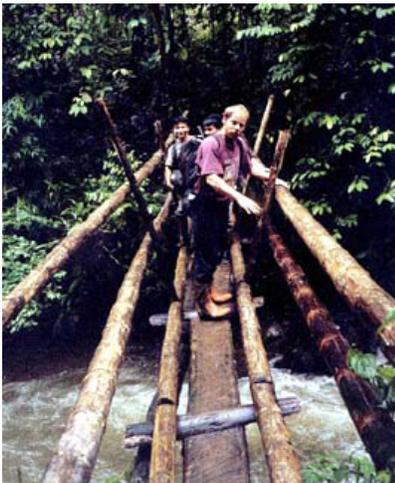
**Figure 16:** Bridges can be constructed from local materials and need not be major structures if equipment can be moved by hand as in this example from Central America. © Energold
