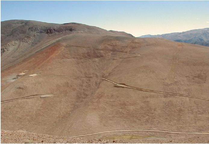
**Figure 27:** Drill roads and on upper left, old trench, Atacama Desert, Chile. Illustrates very slow recovery of old trenches in very arid environment. Also clear is the very visual and permanent effect of roads in this environment. (Photo courtesy Noranda 2004)
