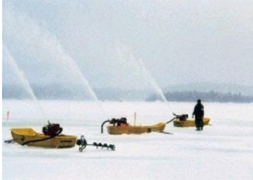
Figure 60: Building the ice pads on Windy Lake. © Wallbridge
