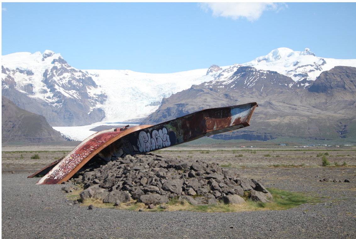
Figure 18: Route 1 bridge destroyed by the 1996 jokulhlaup.
