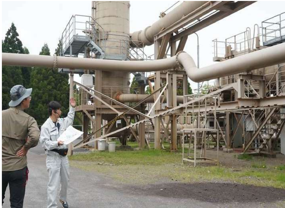
Figure 14: Guided tour of the well, condensation facilities and pipes at the production site.
